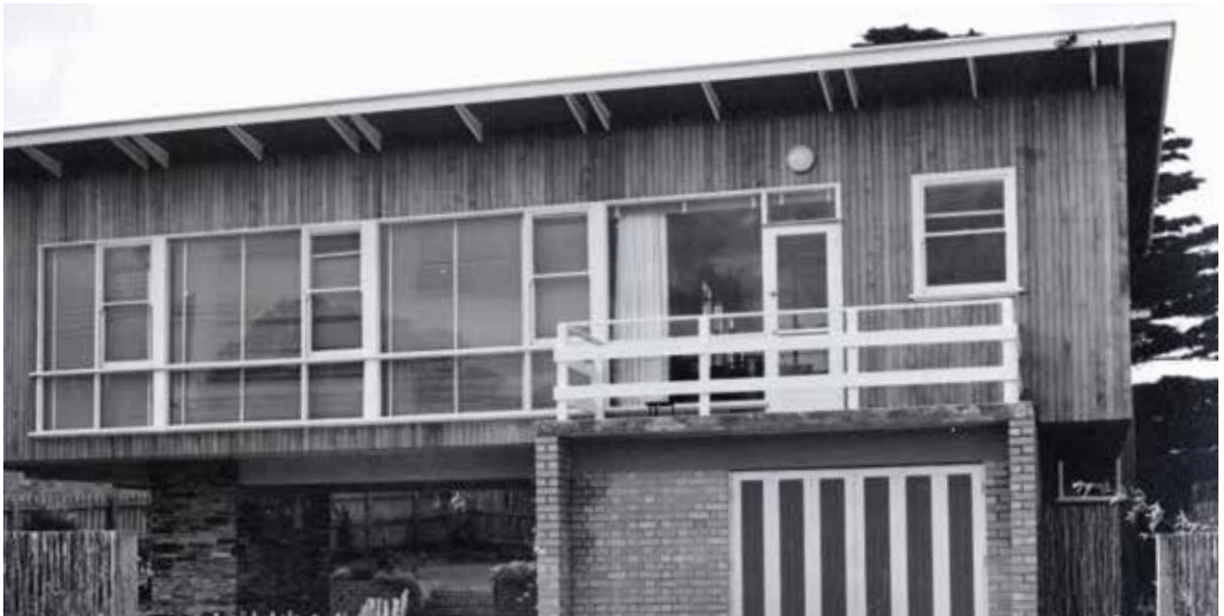
Timber and brick veneer home erected at Beaumaris, Victoria, in 1954 by the War Service Homes Division, Victoria [Homes Erected by War Service Homes Division, Victoria, June 1955]
