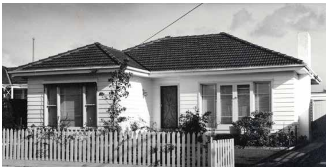
Timber-framed home erected by the War Service Homes Division, Victoria, in 1952 at East Brighton [Homes Erected by War Service Homes Division, Victoria, June 1955]
